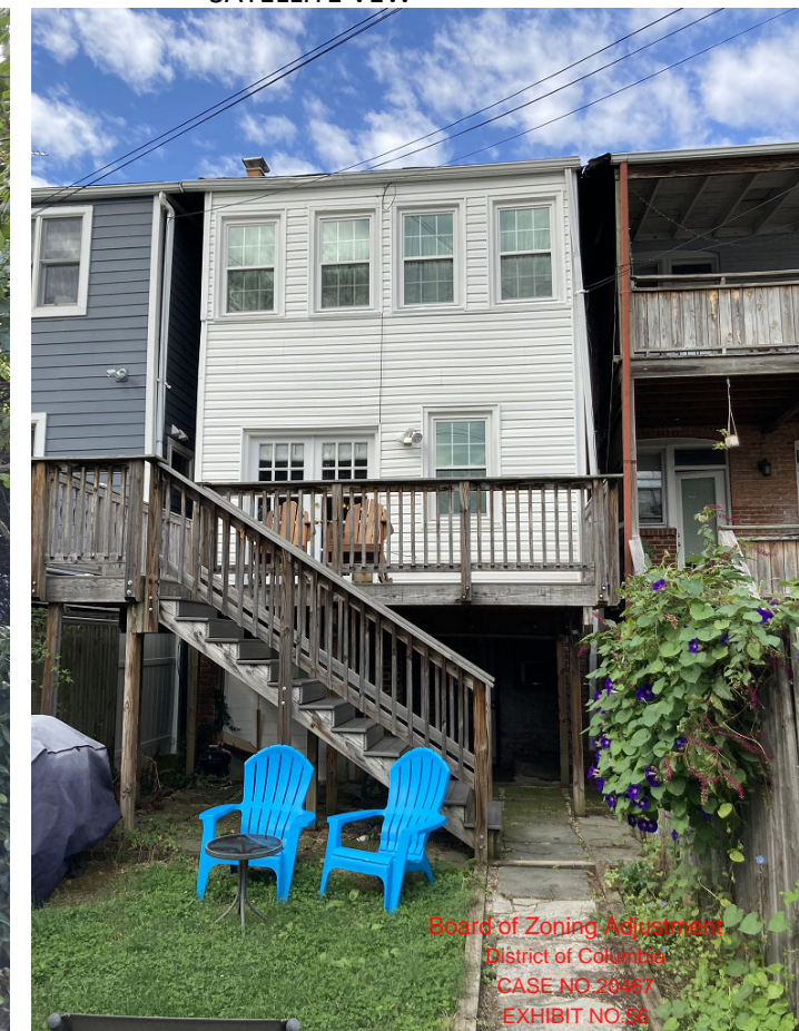
EXISTING REAR FACADE
